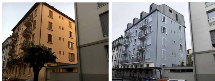
Figure 2: North and East façade before and after refurbishment
